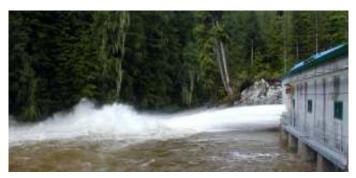
Fig.1: Valve discharge at 15% opening of the valve.
